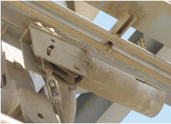
PT&P Hot-dipped Galvanized Support 25 Years In-Service in Dubai - Salt Air from Persian Gulf - 100 Sandstorms per Year
