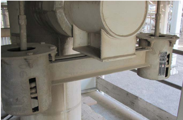
PT&P Hot-dipped Galvanized Support 25 Years In-Service
